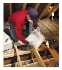
Recycled products can even be used to keep your house warm this fall. Use old glass bottles to insulate your home! Fiberglass Insulation is 25% to 40% post consumer recycled glass.
